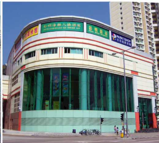
將軍澳彩明商場是首幢符合「成效為本建築物能源效益守則」的建築物。 The first certificate certifying compliance with the performance-based code was issued for the Choi Ming Shopping Centre in Tseung Kwan O.
