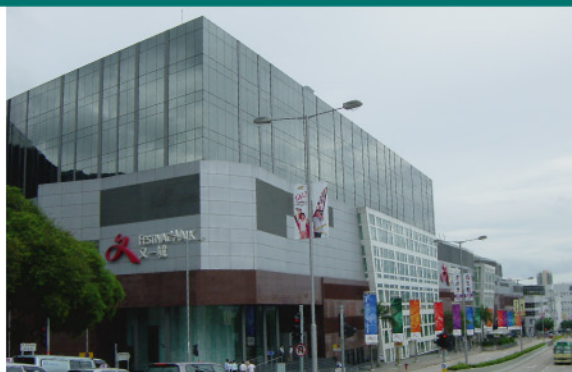
又一城用了水塔，每年節約超過四百萬度電 At Festival Walk, over 4 million kWh saved each year using cooling towers
